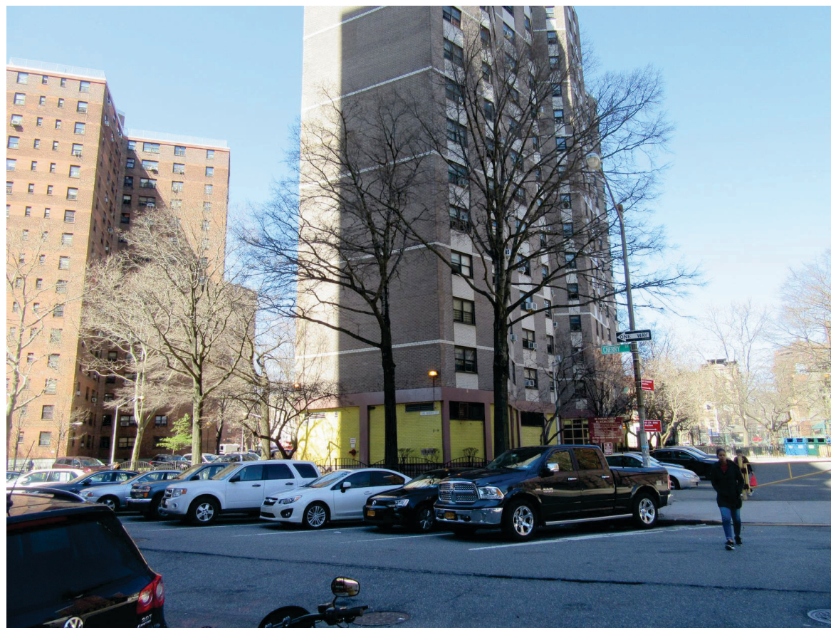
12. View of the north side of Cherry Street between Rutgers Street and Jefferson Street facing northwest.
