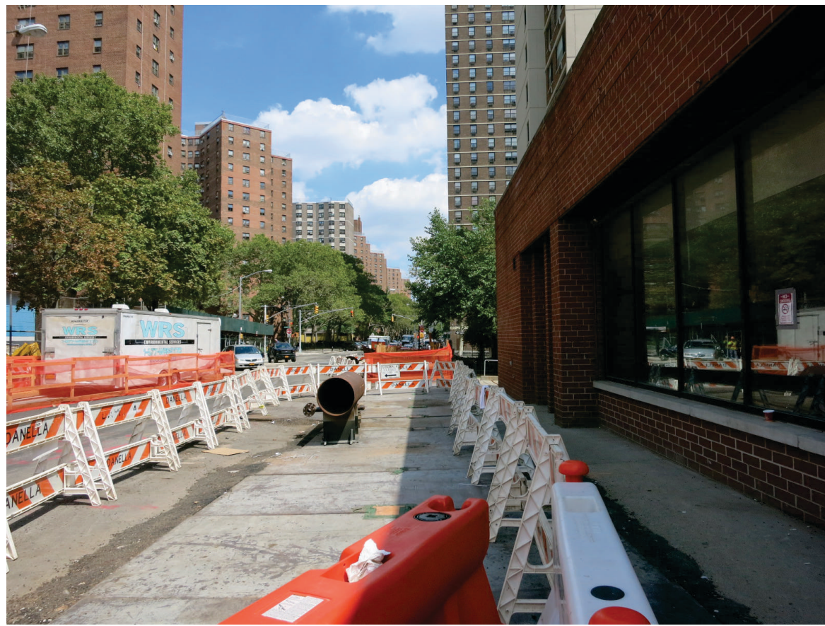
7. View of the sidewalk along the south side of Cherry Street facing east (Parcel 4A at right).
