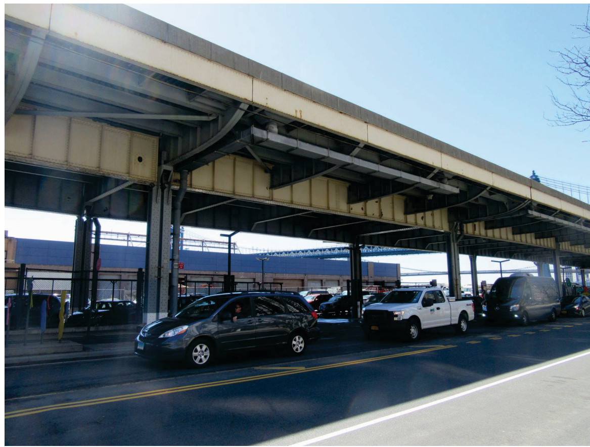
19. View of the south side of South Street and the FDR Drive facing southwest.
